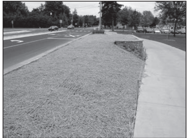
An area at finished grade that has been seeded and mulched.
