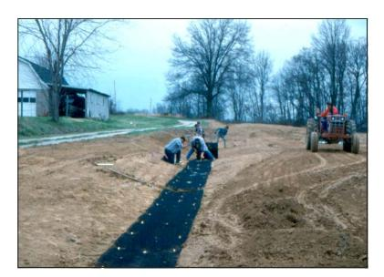
A turf reinforcement mat is a three-dimensional matrix of polypropylene, nylon, or other material typically used in channel applications or on slopes to reinforce plant rooting systems and the underlying soil material.
