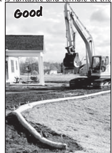
House with straw wattles in place
