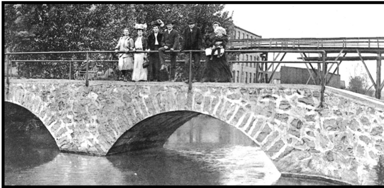
This close-up is of the Jefferson Street stone arch bridge over the millrace. It was built in 1904 for the Hawks Furniture Co. The bridge was also a great help to citizens walking to Tonawanda park and later to Island Park to see baseball games.
