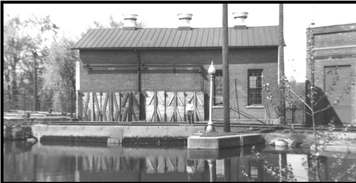
The picture at left shows the power house and the intake gates where the water entered and dropped 14 feet through the turbines to river level.
